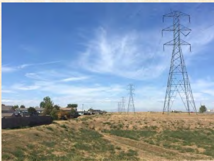
Trail potential adjacent to canals and within utility corridors
